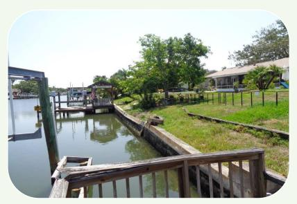
Another vulnerability of grey infrastructure is that it does not traditionally have any mechanisms for adaptation or flexibility, and it has a definite lifespan. The seawall in this photograph likely failed due to a combination of wave action, storm surge, and outward pressure from the upland. There was no vegetation on the waterside of the wall to help break wave action, nor was there vegetation on the landward side of the wall to help stabilize soils.
